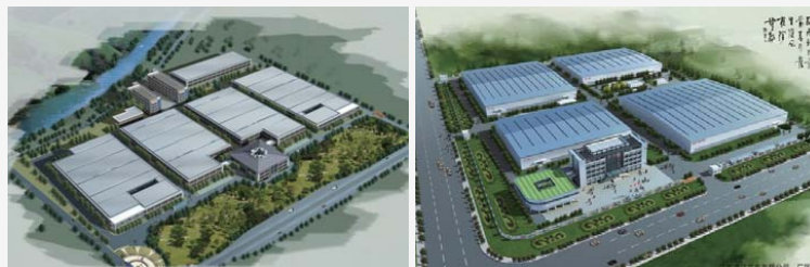
Under construction 2008 new facility
